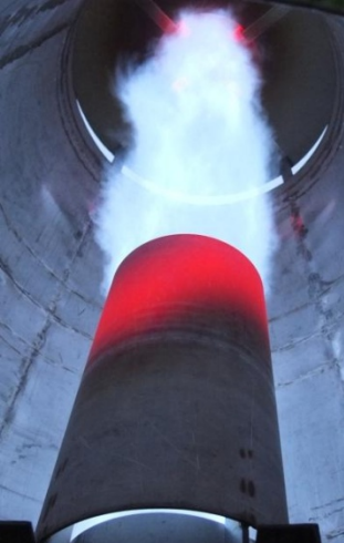
Clean gas burner
